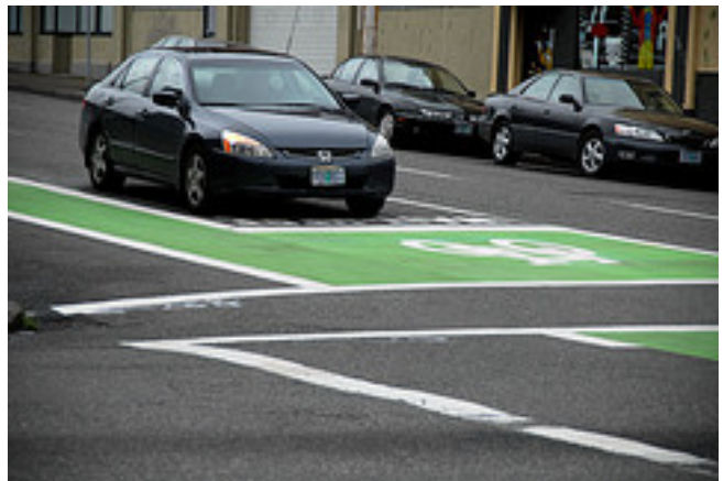
Portland's "bike boxes" are a new roadway engineering treatment being used to improve bike safety at intersections. They are intended to improve awareness and visibility of cyclists and to help prevent dangerous "right-hook" collisions. Photo courtesy of BikePortland.org.
