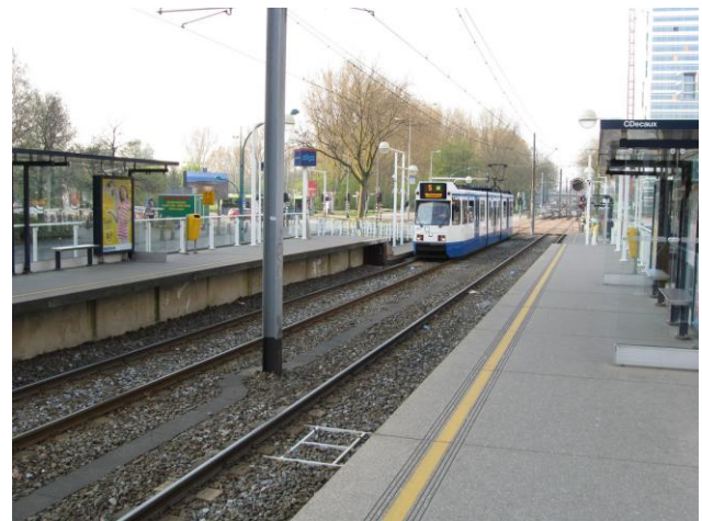
Figure 7. Split level platform in Amsterdam, Netherlands allows transfers between high-floor metro (LRT) trains and low-floor trams using the same track (photo: Daniel Sparing)
