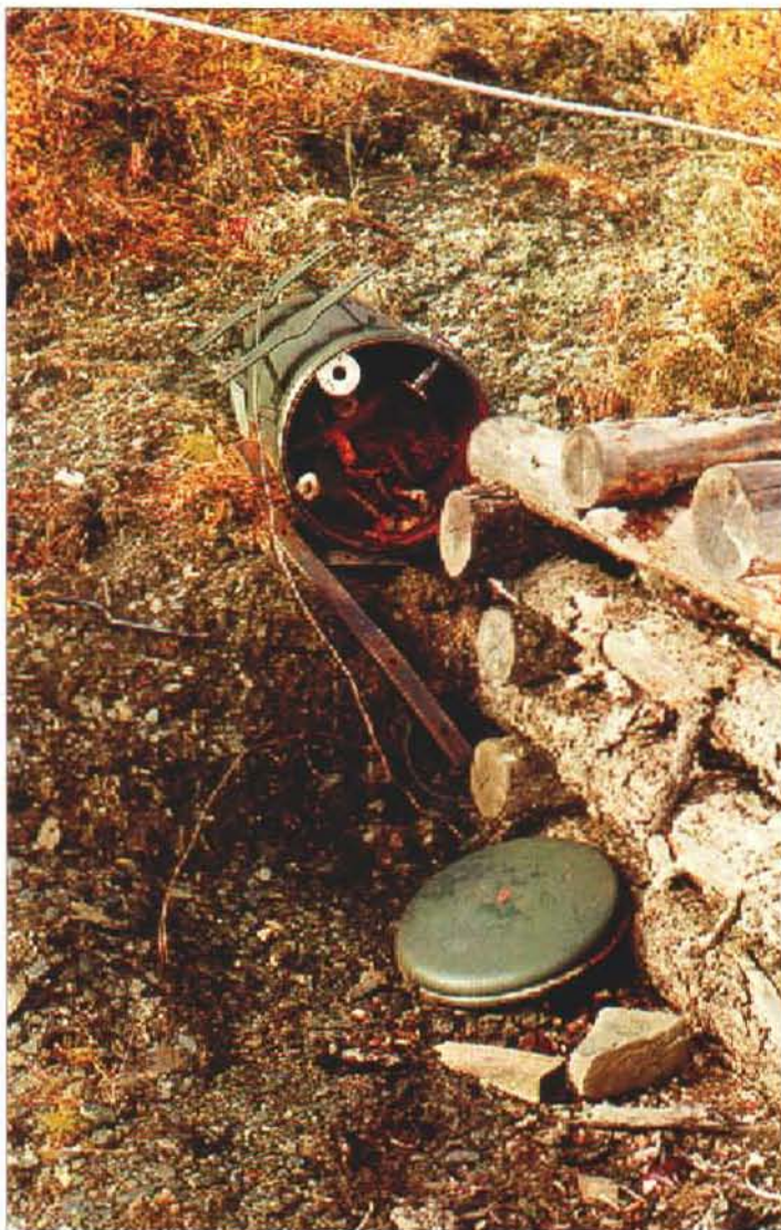
Photo 32-26 : Keno 200. Fallen capacitor / transformer by tower.
