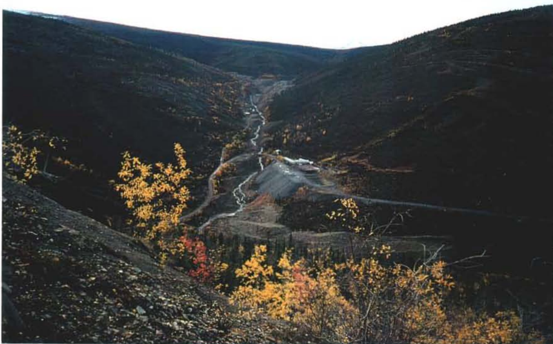
Photo 22-20 : Overview of Bellekeno site. Note use of mine waste rock for road ballast and its proximity to creek in Thunder Gulch.(Azimuth 170°)
