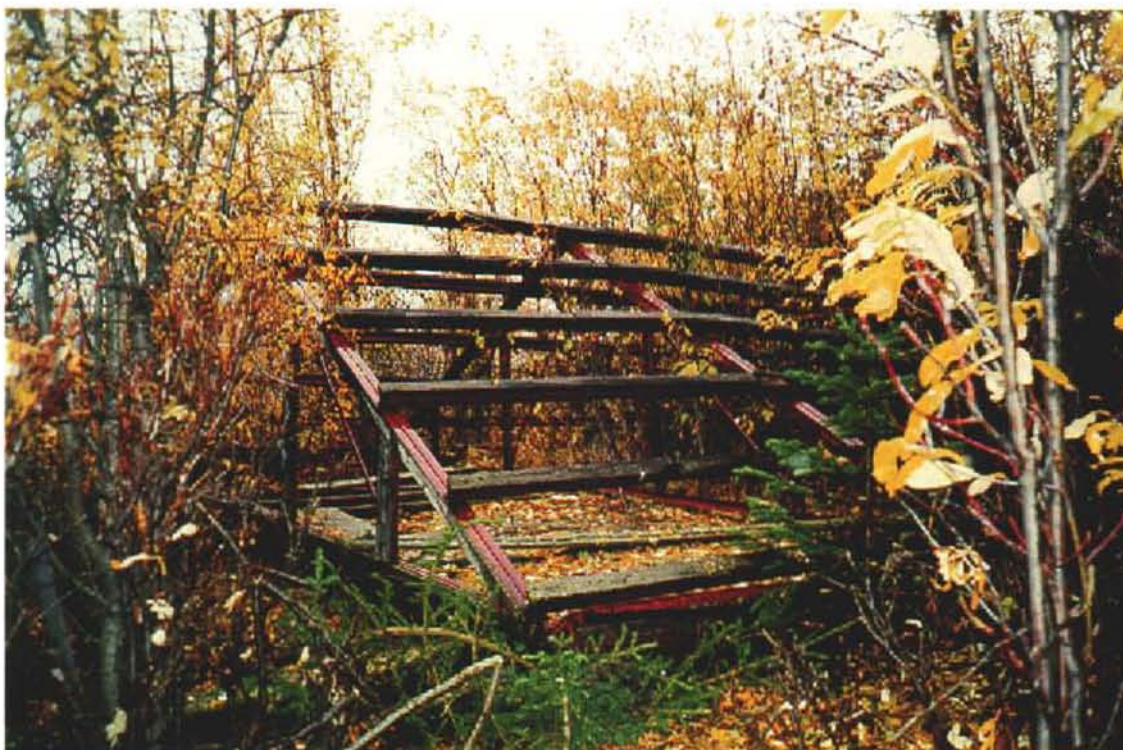
Photo 27-6: Collapsed steel building frame (Bldg. 27-2). (Azimuth 120°)
