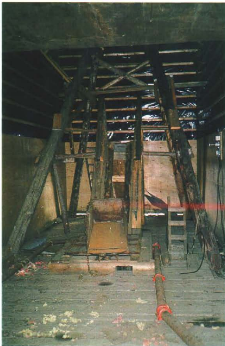
Photo 26-7: Interior of Lucky Queen headframe building (Bldg. 26-A) showing open manway and boarded shaft opening.
