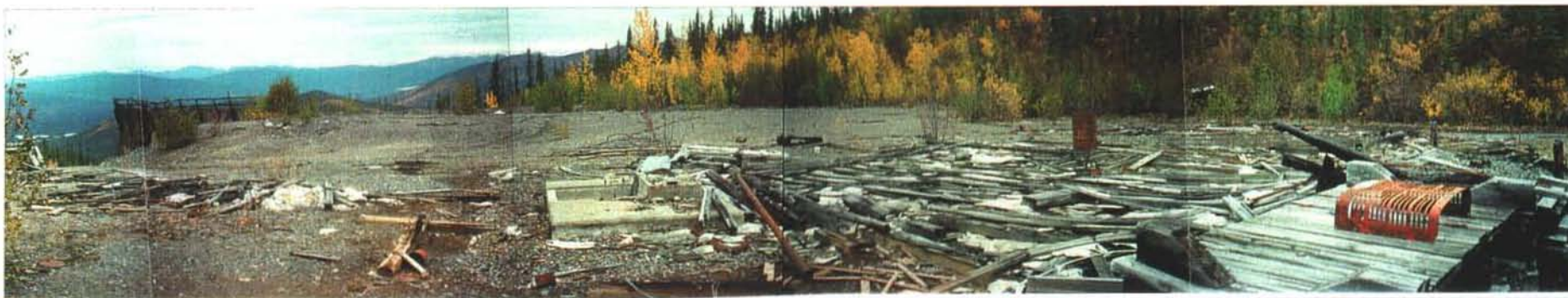
Photo 21-1: Panorama of main Werecke Camp and Sadie Ladue Mine area showing end dumped waste rock and overburden piles, Pitt#1 and decline hole to left, and partially collapsed shaft structures to far right.
