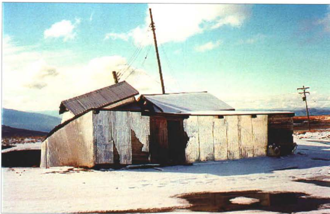
Photo 36-2 : Keno No.9 Shamrock J18 Vein Raise Building (36-A). Note collapse of building into failing underground workings and fencing around opening. Also, transformer on power pole in background. (Azimuth 290°).
