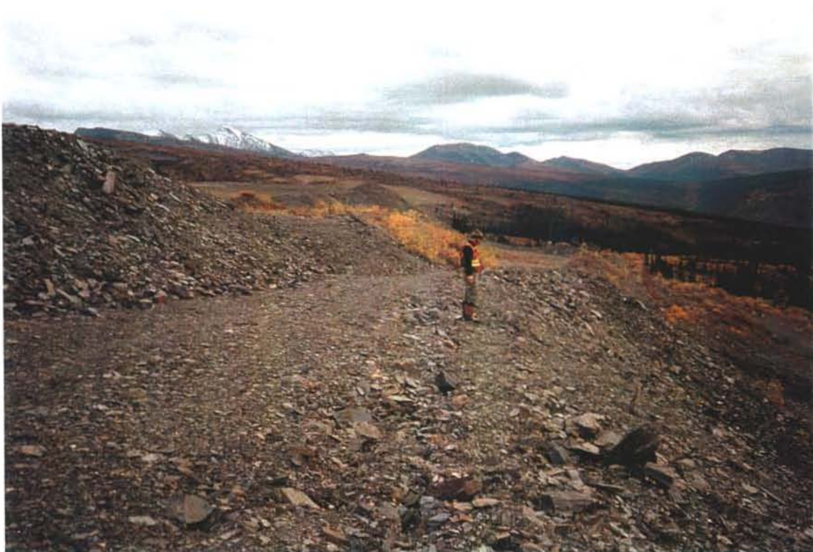
Photo 25-12: Tension cracks on edge of waste rock pile. Note slumped edge running along edge to mapper. (Azimuth 180°)
