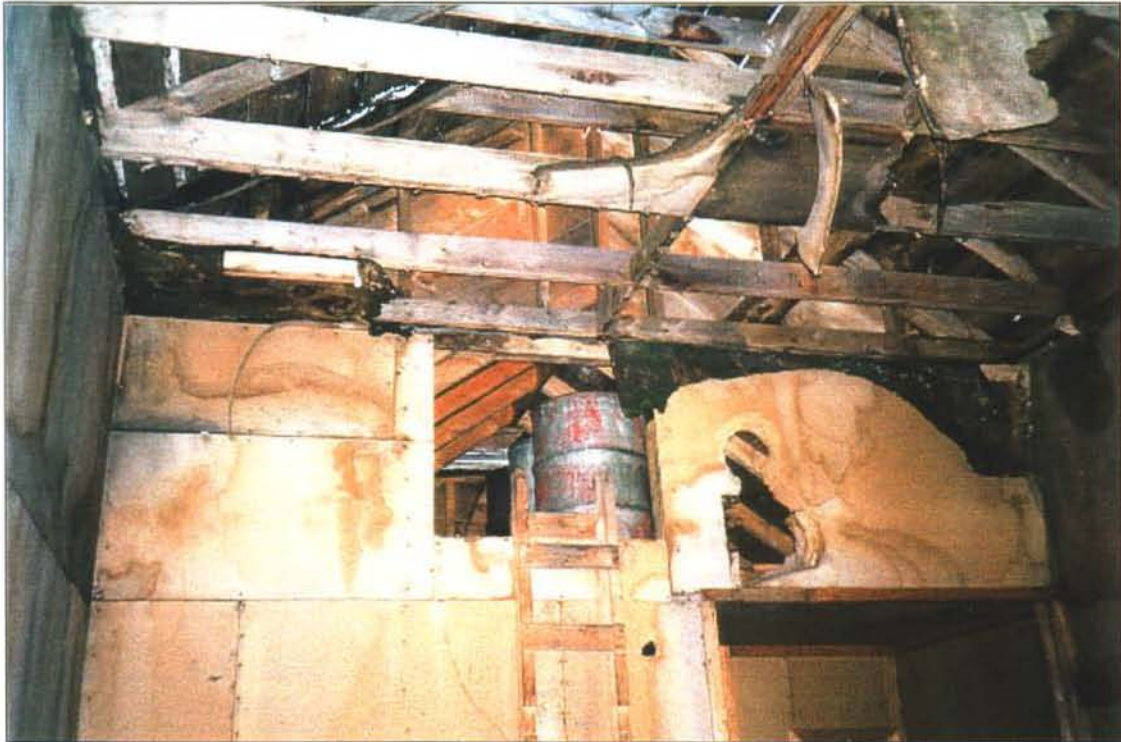
Photo 31-7: Interior of dry (Bldg 31-A) showing rafters, wallboard and water tanks for shower and sauna.
