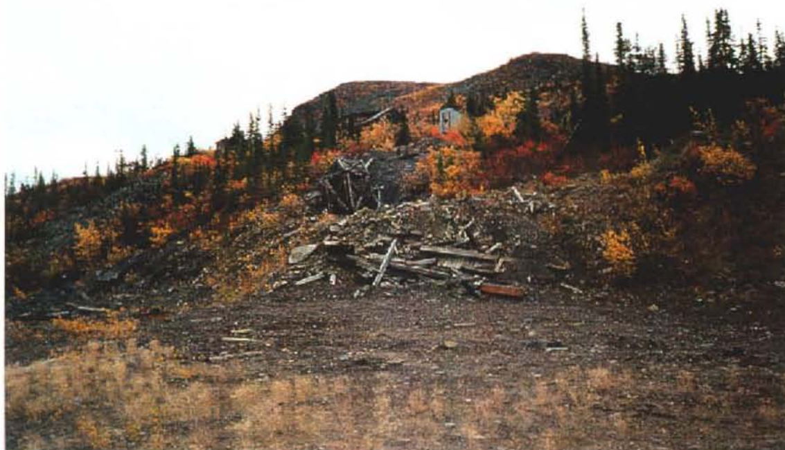
Photo 21-4: Sadie Ladue shaft area. Note dilapidated tressel, outhouse over callapsed manway and managers house in background. (Azimuth 080°)
