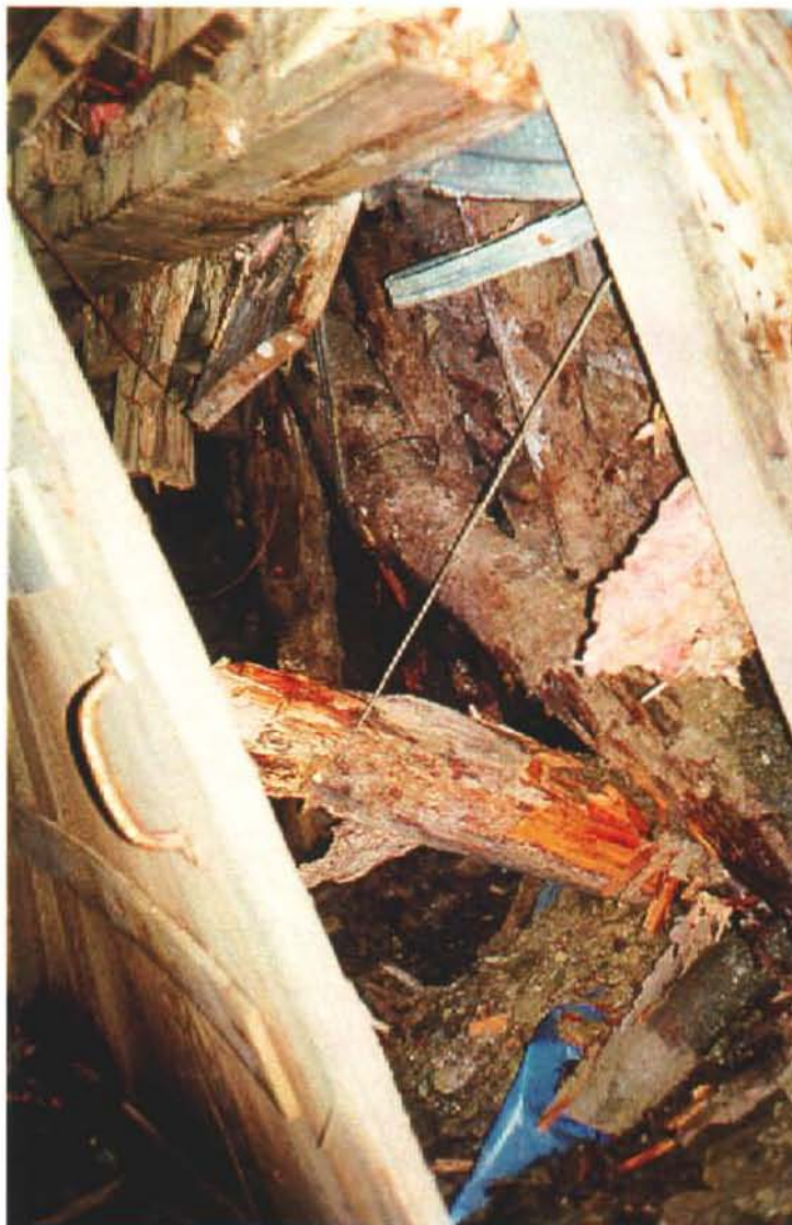
Photo 25-9: Collapsed portal timbers behind door.
