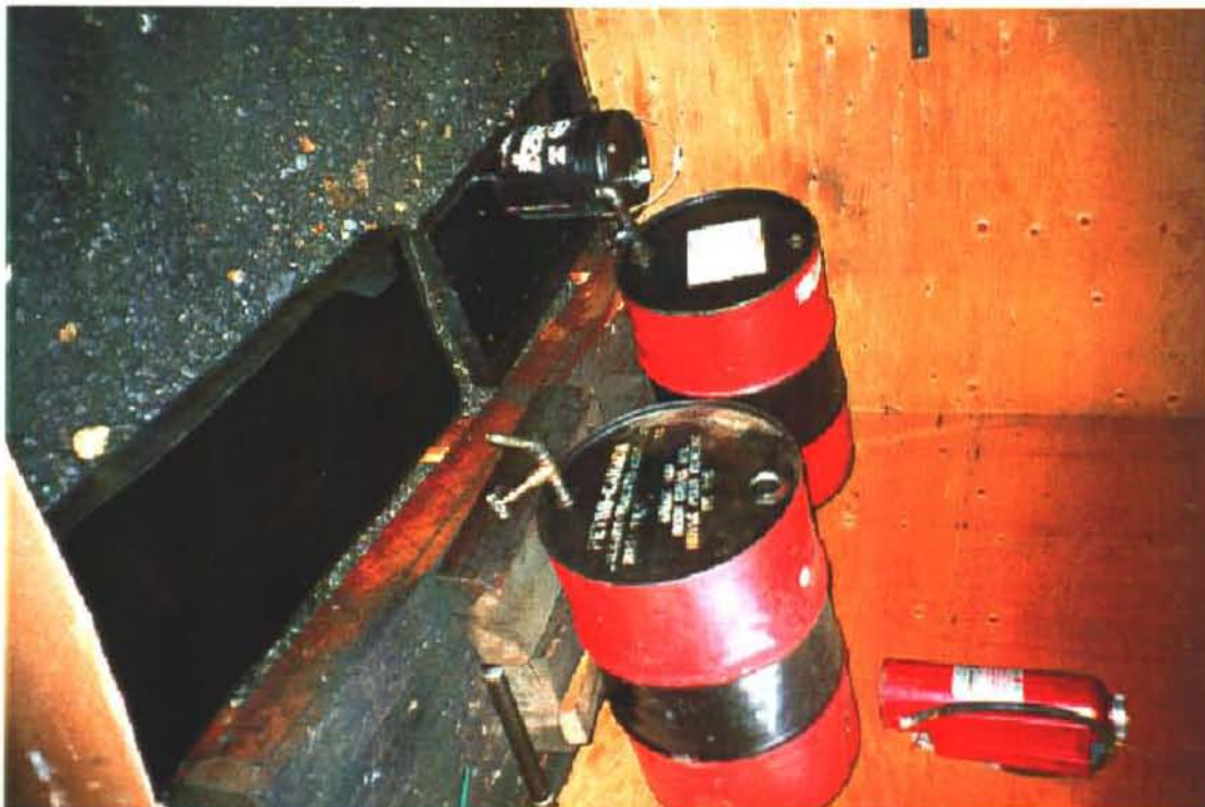
Photo 22-6: Oil barrels fitted with dispensing valves located inside compressor house. Spill trays are filled with oil and hydrocarbon staining is evident on floor.
