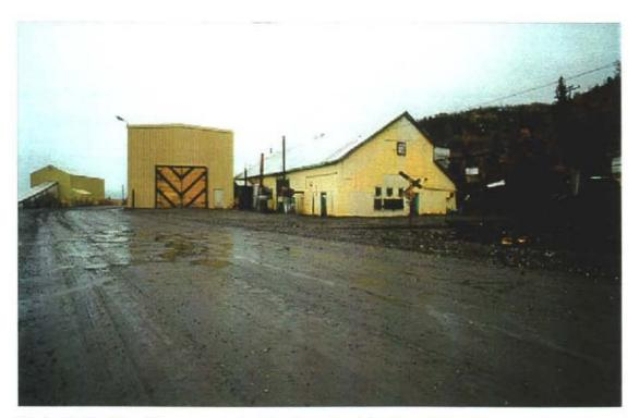
Photo 78-28: Elsa. The generator building is on the right, the vehicle & heavy equipment warehouse is in the centre, and the building in the background is the crusher house. The 3 diesel exhaust stacks are visible on the left side of the generator building.
