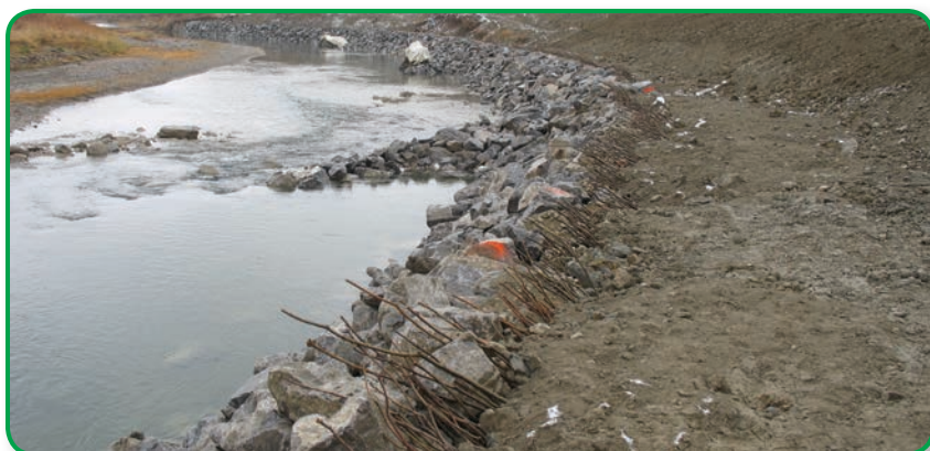
Biotechnical stone toe protection with brush layering.
