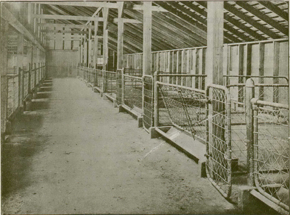
Fig. 29.—Interior view of well lighted Piggery, showing the north row of pens lighted from upper windows.
