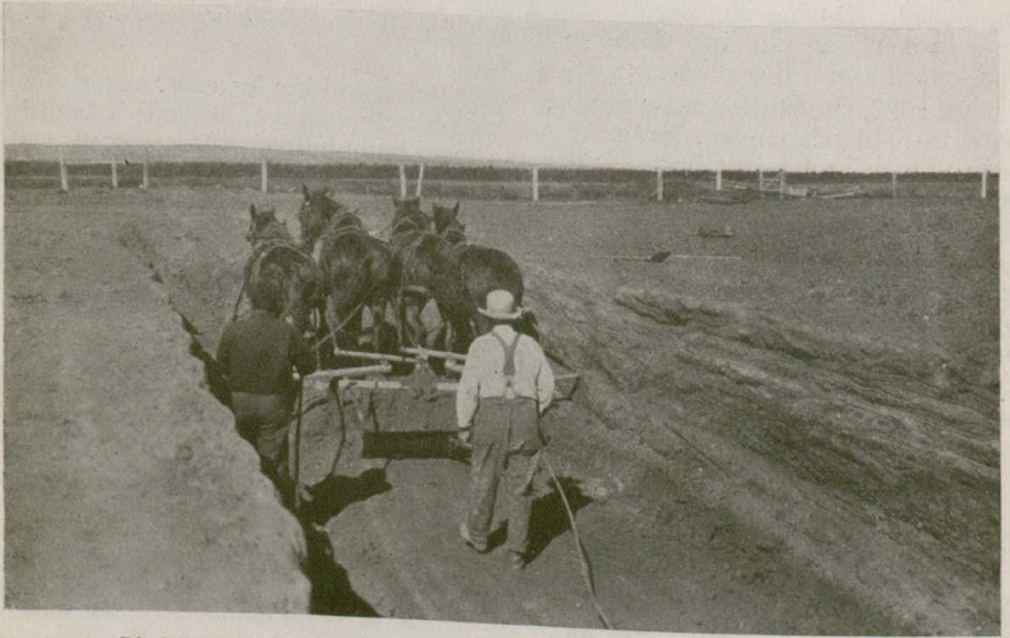
Digging a trench silo (the Fresno saves Time)—Experimental Station Swift Current, Sask.
