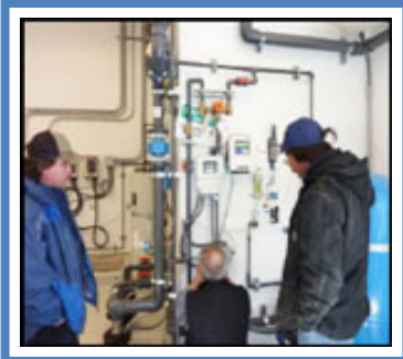
Circuit Rider & Water Treatment Plant Operators performing routine maintenance
