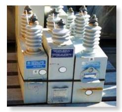
Capacitors are devices that accumulate and store electrical charge and are found both inside and outside buildings. Because capacitors have multiple applications, their size, shape and appearance may vary. They may be mounted on panels, in boxes, on walls or on floors, individually or in banks.
