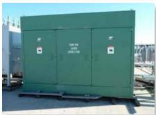
**Transformers** take electricity of one voltage and change it to another voltage. They are widely used and found in a variety of locations. Transformers that use a liquid coolant, or "wet" transformers, may contain PCBs. Dry-type transformers will have air vents for cooling and do not contain PCBs.
