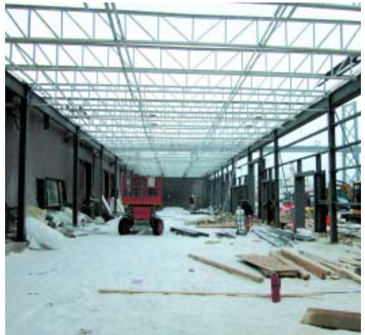
Vulcan Building construction
