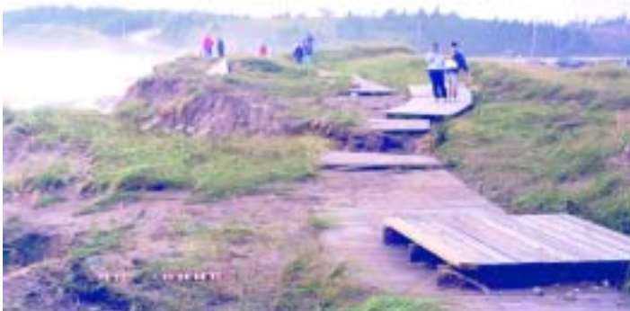
Erosion and damage at Lawrencetown Beach caused by Hurricane Juan – photo by Bob Taylor
