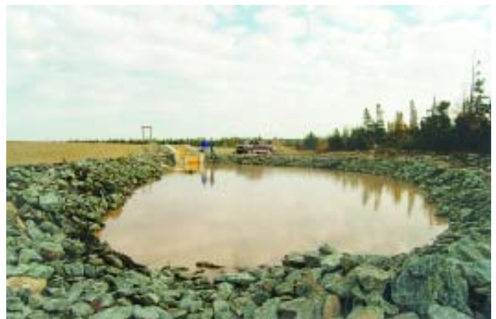
The headwater reservoir which is the source of cold water for the siphon - photo by Bob MacDonald
