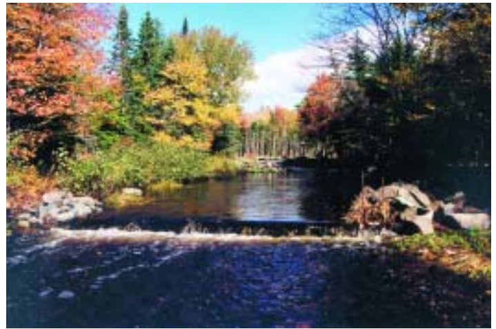
The St. Francis Harbour River after siphon installation, fall 2003 – photo by Jack Ronald
