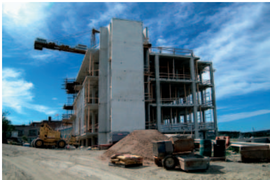
Structural elements of the new lab nearing completion
