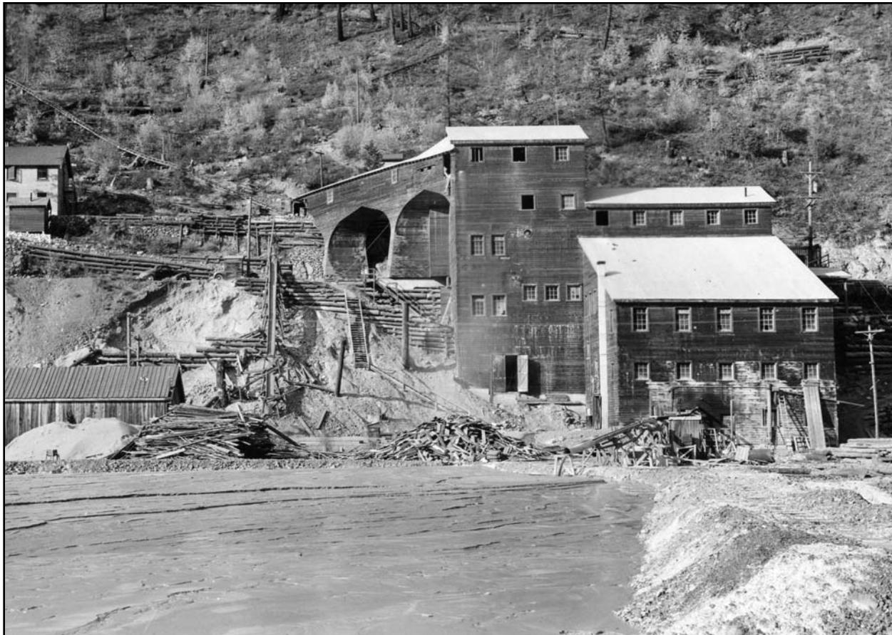
**Fig. 10.** Stamp mill at the Minto Mine in October 1937 (photo by C.E. Cairnes, GSC, No. 82986). The flat area in the lower left part of this photo is a delta composed of sulphide-rich tailings that are actively being deposited into the Bridge River from a sluice extending out of the mill. The remains of this mill are now flooded by Carpenter Lake (Fig. 1). Reproduced with permission from the Natural Resources Canada Photo Database, Ottawa.
