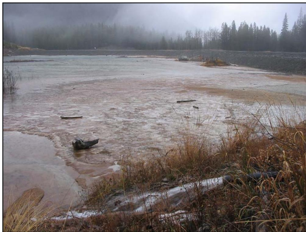
**Fig. 8.** (a) Upwelling point in the underground workings at the Bralorne Mine, where As-rich water rises from the flooded mine workings before discharging at the 800-Level portal. (b) Mine water from 800-Level portal (Fig. 7a) being discharged into the Bralorne tailings impoundment.
