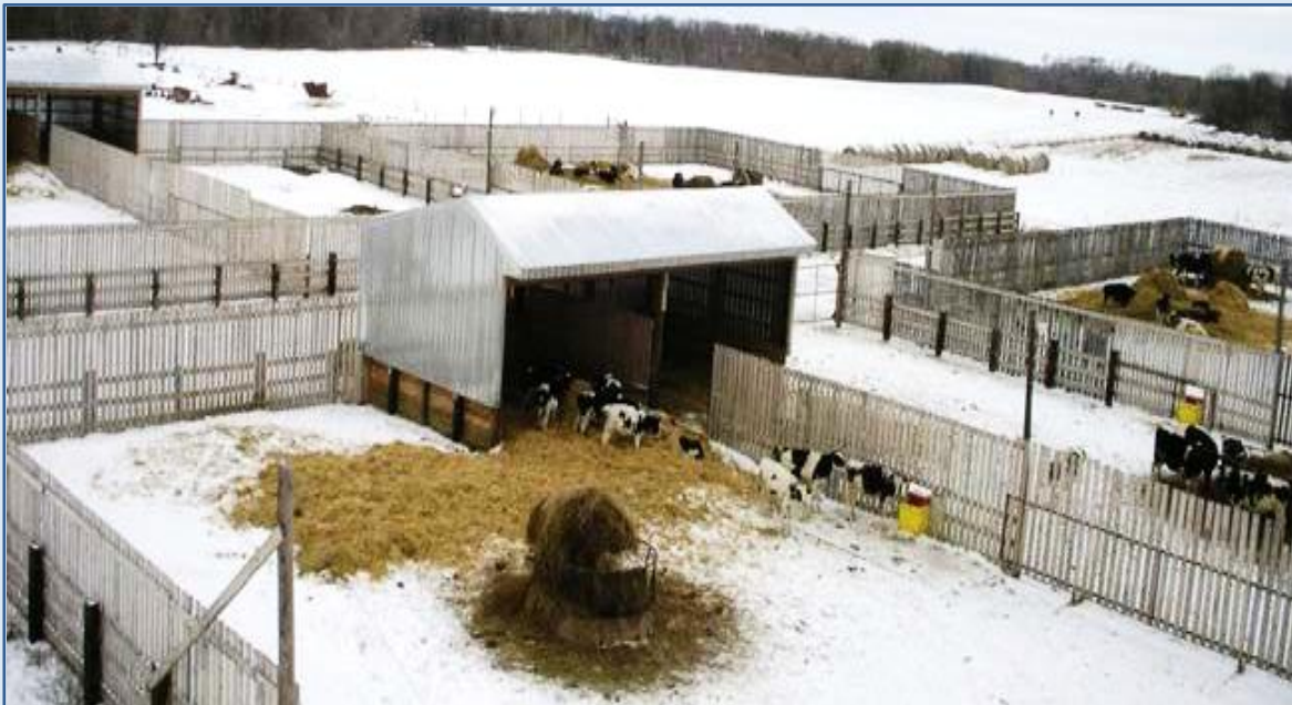
Vuignier's newly constructed pens on the new site with sufficient distance from the creek
