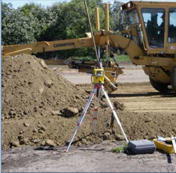
Pen floor construction required surveying and laying of a surface clay foundation
