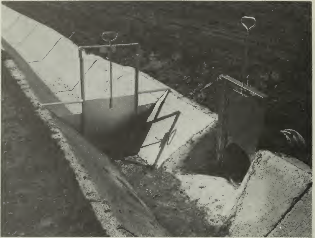
Fig. 7. Concrete lining installed in drainage canal.
