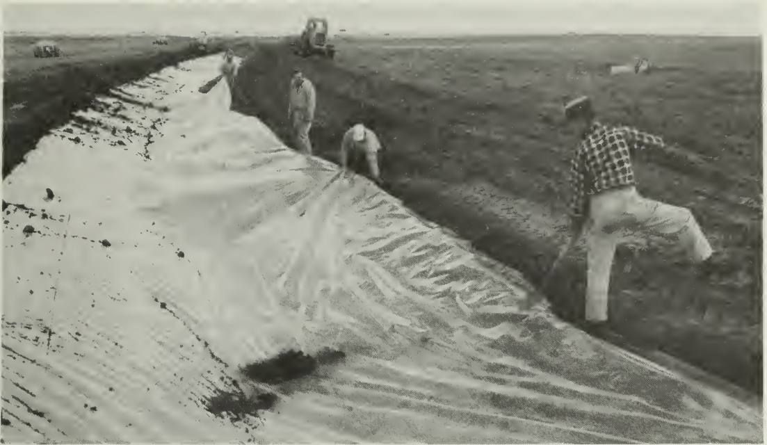
Fig. 9. Installing plastic lining, which will be covered with soil for protection.
