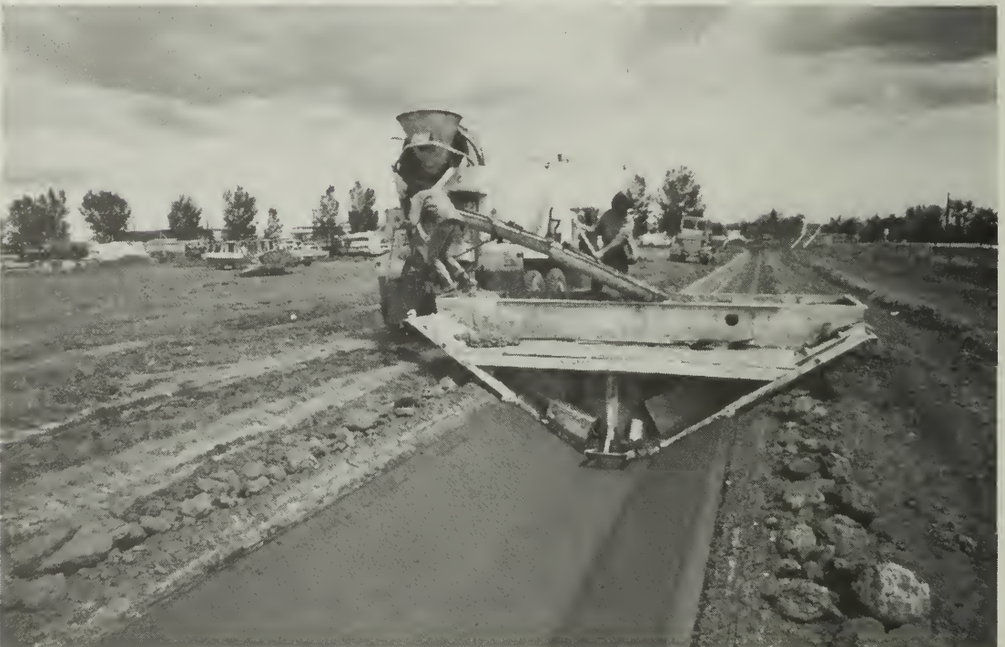
Fig. 8. Slip form used to install concrete lining.
