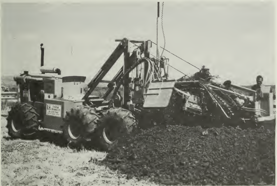
Fig. 12. Wheel trencher for installing subsurface drains.
