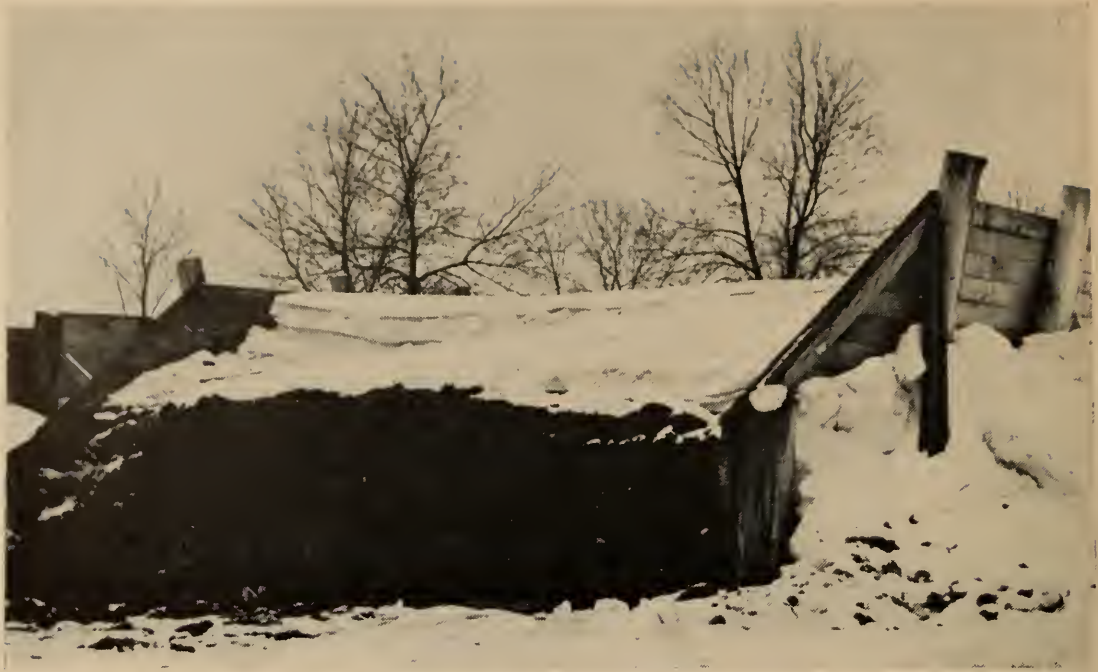
Figure 2. A horizontal silo is a relatively cheap means of storing grass silage.
