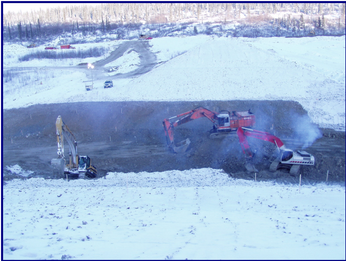
Soil excavation at Faro Mine
