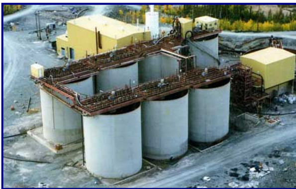
Tailings reprocessing plant at Giant Mine
