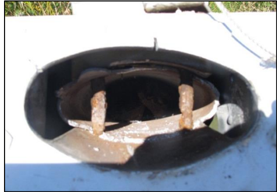
Photo 5. Corroded through-bolts
