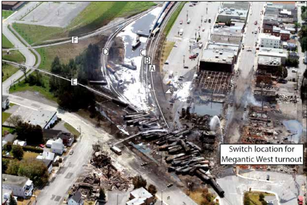
Photo 5. Eastward view of the location of the tracks in relation to the first derailed cars: main track (A), yard track 1 (B), yard track 2 (C), yard track 3 (D), and the west and east legs of the wye tracks (E and F)
