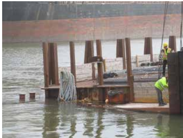
Photo 4. After end of barge during loading
