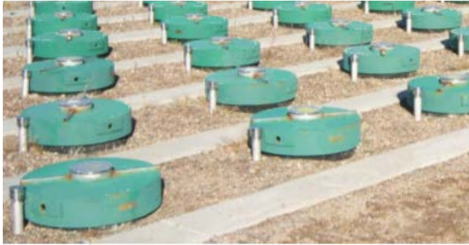
FIGURE 2: Tile hole storage for cemented Mo-99 waste.
