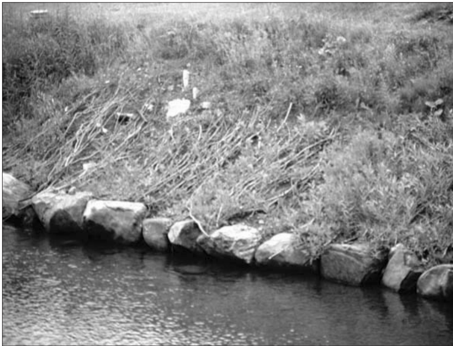
Example of bio-engineering to stabilize eroding shoreline. Photo: Denis Lehoux, Environment Canada
