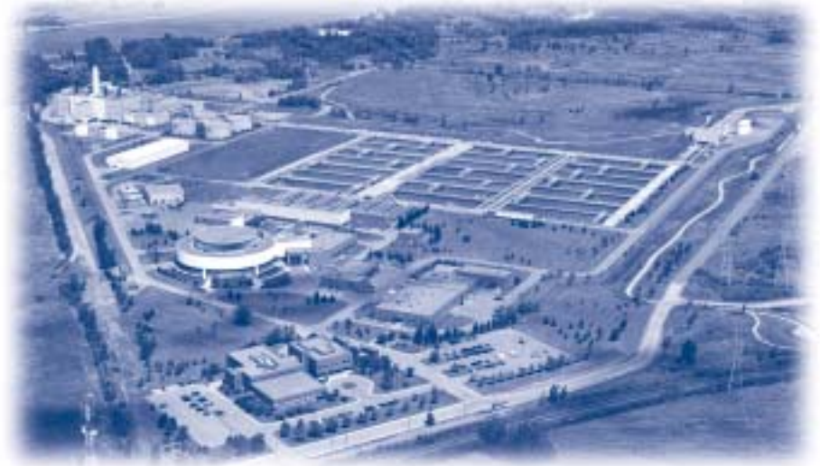
Montreal Urban Community (MUC) wastewater treatment plant Photo : MUC
