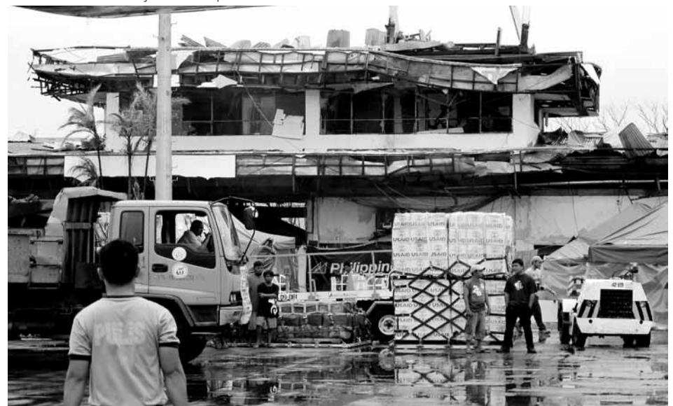
The airport at Tacloban was heavily damaged by the typhoon. Local authorities, the military and available support teams cleared the runway to secure a path for relief efforts.
