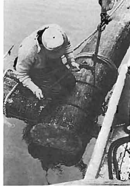
Plate 2-6. Cable being tightened at corner.
