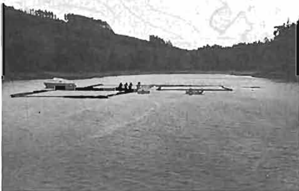
Plate 2-2. Pond site Parson Bay. Pond No. 1 (b) being installed.
