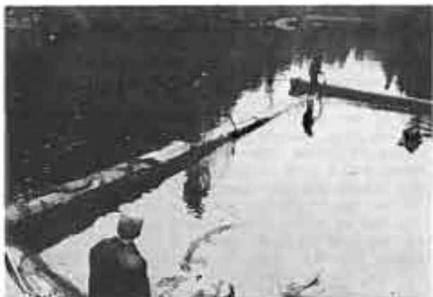
Plate 2-8. Edge of web being nailed or stapled to logs.
