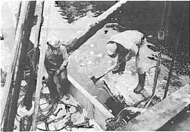
Plate 2-4. Notching the ends of logs.
