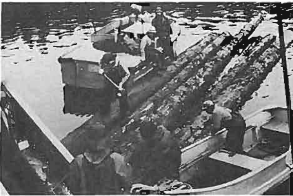
Plate 1-1. Log bundle. A bundle of cedar logs is being unbundled preparatory to pond construction.
