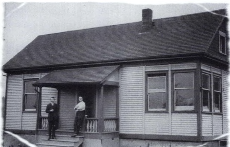
Alert Bay, VAF, in the very beginning. Operator Jack Bowerman (left) standing next to an unidentified operator, 1913. (Richard Loeb)
