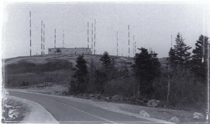
Transmitter building at Halifax Coast Guard Radio VCS, Pennant, 1980. (John Rae and Paul Britton)
