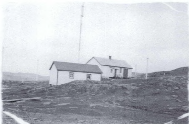
Outside view of Marconi station at Belle Isle. The longer building housed the radio station. The four short masts supported the direction-finding loops. The longer mast in the centre supported the main antenna, 1956. (Samuel Johnson)
