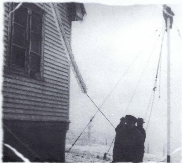
Camperdown staff repairing antennae after an ice storm, 1938. (W.H. Wooding)
