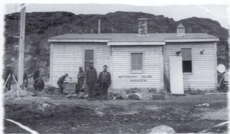
The Northwest Territories' Nottingham Island, VCB, station under construction, 1927. (National Archives of Canada, PA55537)
