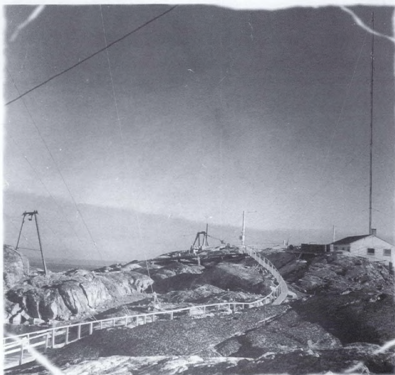
The radio station at Resolution Island, Northwest Territories, with its inverted "V" antennae. The highest tower on the right is the low-frequency antenna and the shortest is the high-frequency antenna, 1960. (Raymond Douville)
