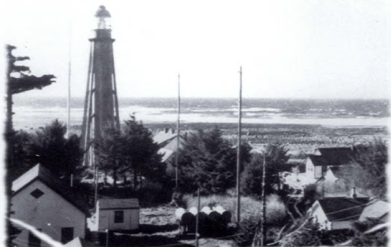
The Estevan Point station, VAE, on its perch on the west coast of Vancouver Island. During World War II, the lighthouse and nearby buildings were fired on by a Japanese submarine, the first attack on Canadian soil since the War of 1812. Material damage was incurred, but no lives were lost, c. 1950. (Courtesy of the S.P.A.R.C. Museum)
