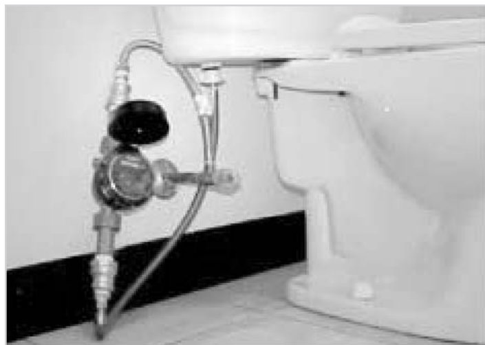
Figure 3 Inline water meter for measuring flush volumes
