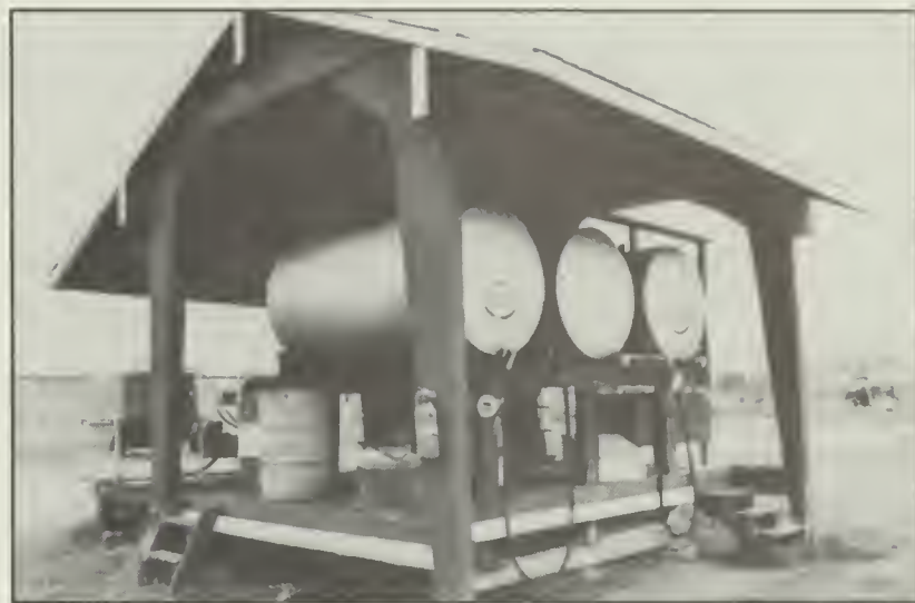
Fig. 2.12 b) Light Colors, Shading and Pressure Relief Valves Reduce Evaporation Losses.
