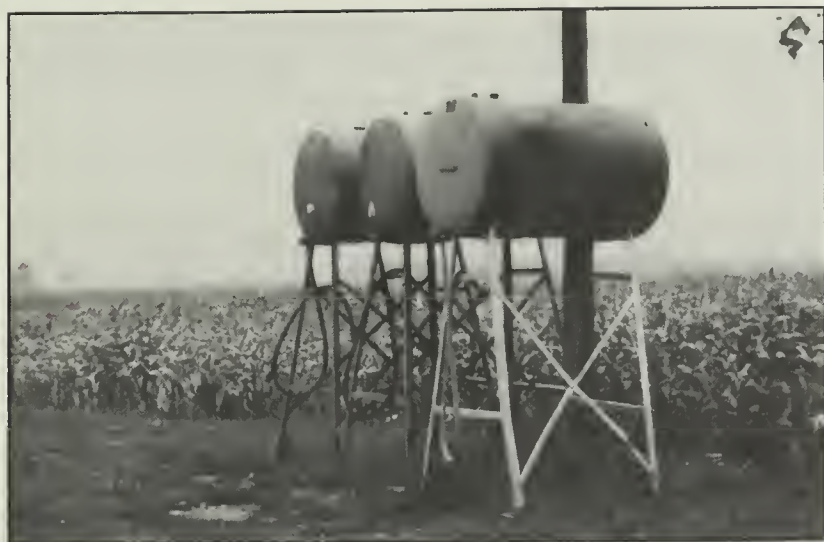
Fig. 2.12 a) Evaporation Losses are Highest from Dark-colored Exposed Gasoline Tanks.
