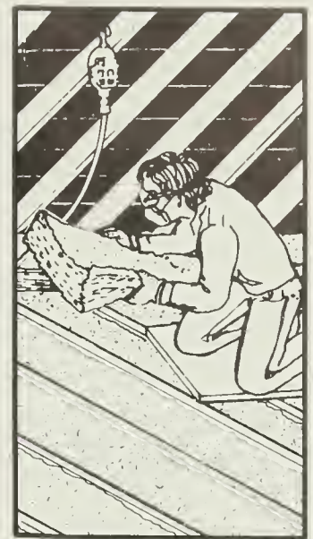
Fig. 3.7 Installing Blanket Insulation in Unheated Attic
