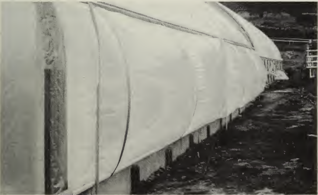
Fig. 9. An inflated polyethylene sidewall ventilator closed with a tight seal.
