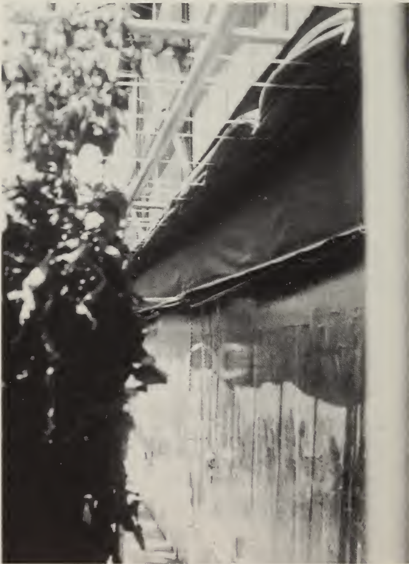
Fig. 12. An insulated north wall in a shed-type greenhouse. The solar-collecting panels, which are suspended from a scroll, are retracted to reflect light.
