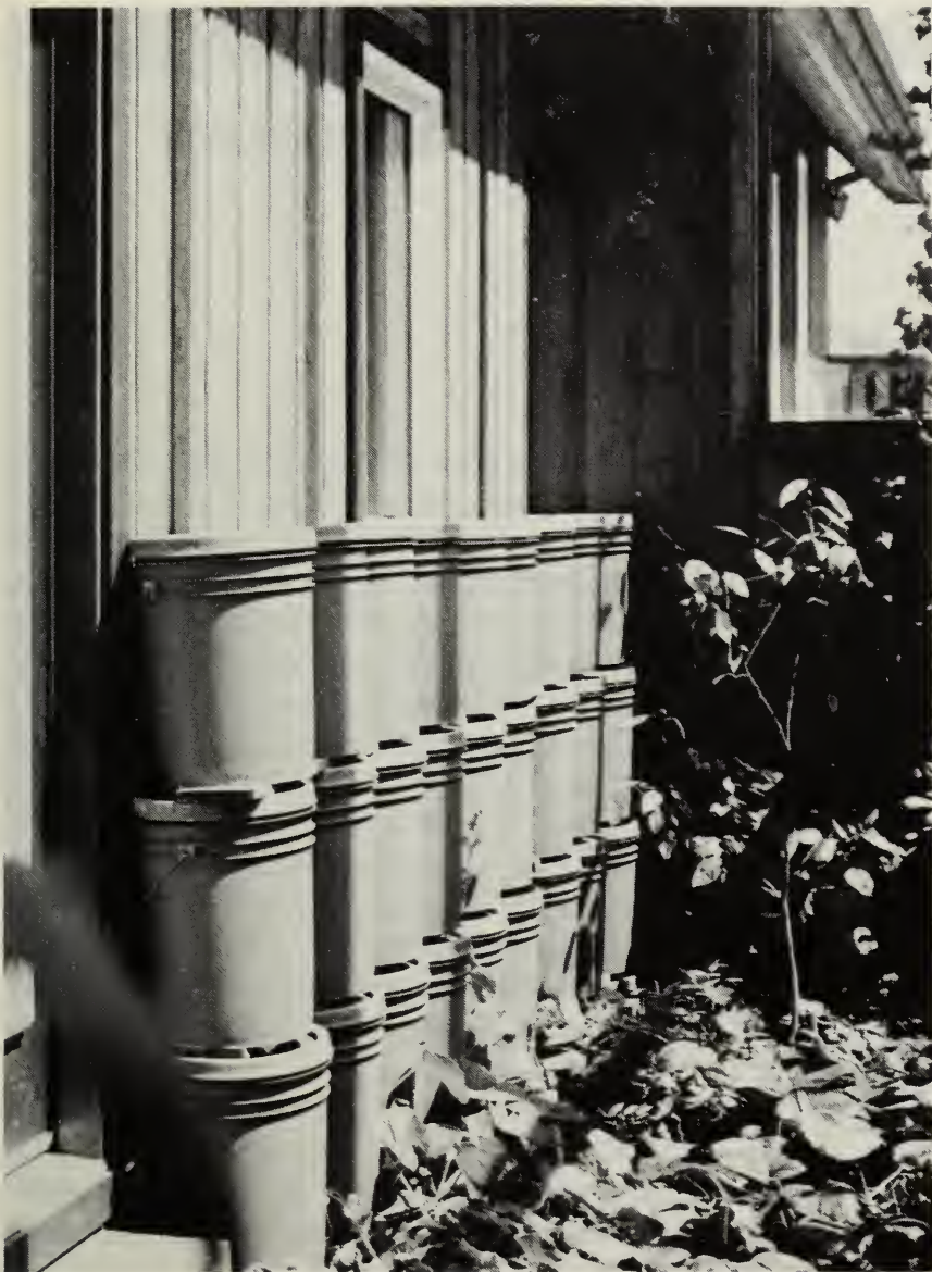
Fig. 17. Water barrels that are used as heat storage in a small greenhouse.
