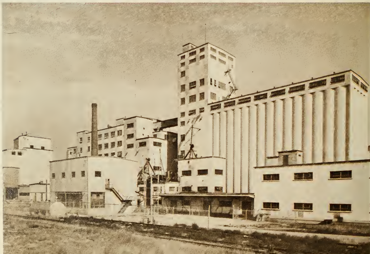
A modern solvent-extraction plant showing receiving and storage facilities, solvent plant, oil plant and refinery buildings (in background: a large flour mill). Photo courtesy of Saskatchewan Wheat Pool.
