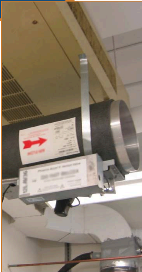
Laboratory room supply air valve
