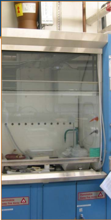
Constant air volume fume hood modified to variable air volume
