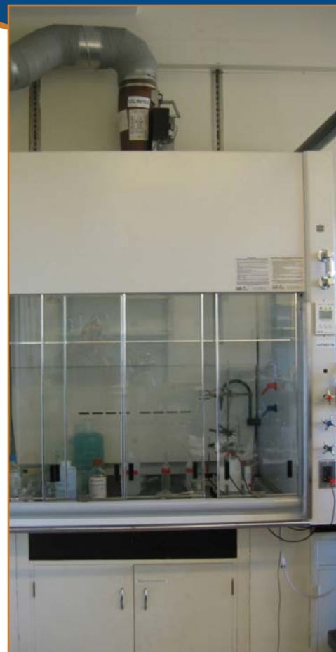
New high efficiency/low airflow fume hood
