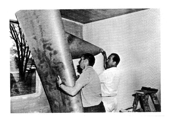
Figure 4-23. The Mark IV house employed a Norwegian system using Kraft paper for the interior wall finish.
