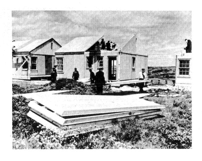
Figure 1-5. This photograph shows installation of prefabricated roofs on wartime houses in Moncton, New Brunswick in 1941.
