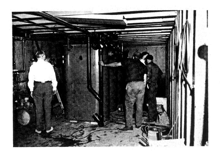
Figure 6-3. This photograph shows the recirculating sewage system used in the Mark IV house.
