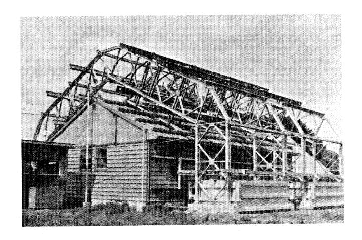
Figure 4-15. In the late 1940s, DBR invented this apparatus to test roof loads.
