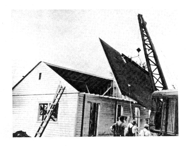
Figure 4-5. This 1941 photograph shows a roof panel being hoisted into place on a wartime house in Moncton, New Brunswick.
