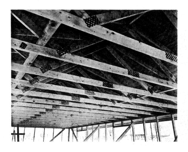
Figure 4-17. Roof trusses, such as these in the Mark IV experimental house in 1964, permitted greater freedom in interior layout because interior partitions were no longer required to support the roof.
