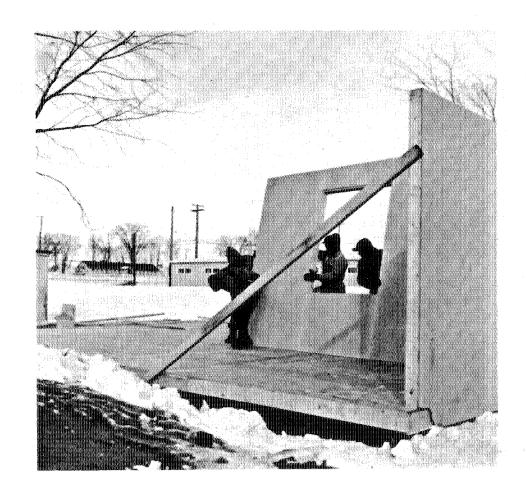
Figure 4-19. Prefabricated panels were used to build the walls of the Mark III house in 1960-61.
