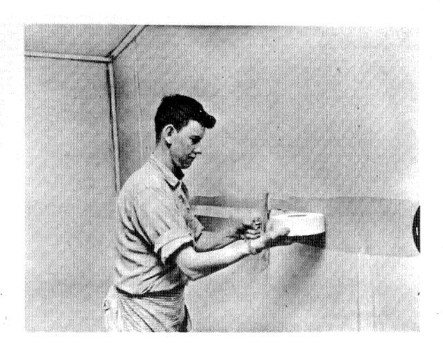
Figure 4-22. Use of sheets of gypsumboard reduced the labour needed for interior finishing. This Ottawa worker in 1960 is taping the joints between the panels.
