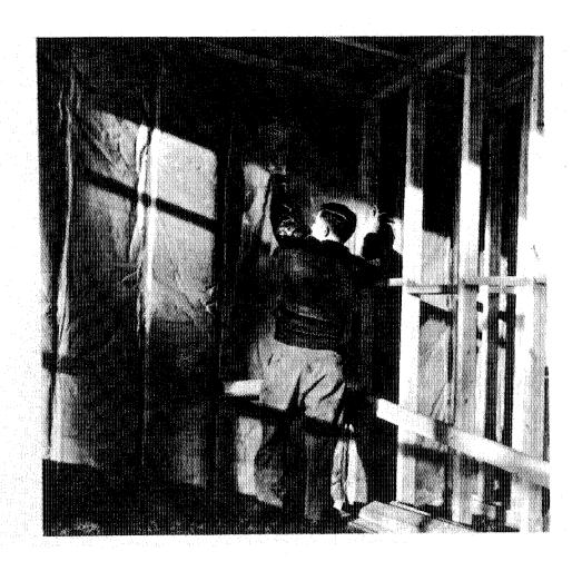
Figure 5-9. Polyethylene vapour barrier, as shown in this 1959 photograph, was in common use in Canada by the late 1950s.
