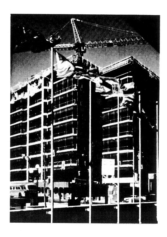
Figure 4-26. The use of climbing cranes and flat slab construction, as on this Ottawa building, revolutionized high rise construction in Canada.
