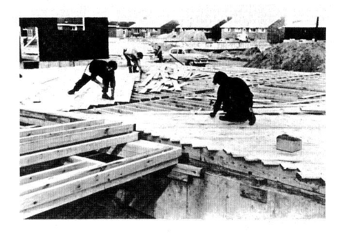
Figure 4-3. This 1958 photograph shows an Ottawa work crew building a floor by nailing boards diagonally across the joists.
