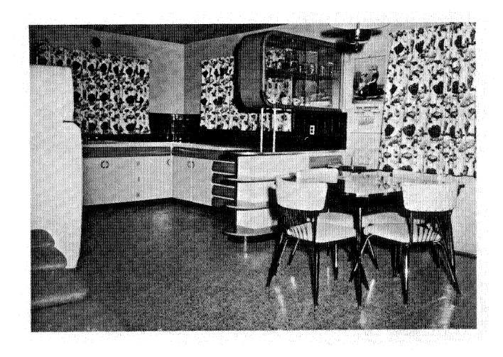
Figure 4-14. By the late 1950s, prefabricated kitchen cabinets, such as these in a Lethbridge, Alberta house, were beginning to replace cabinets built on site.
