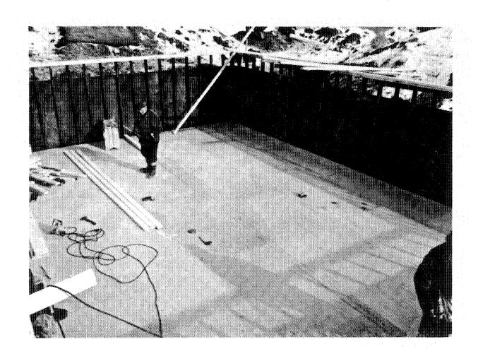
Figure 5-6. The wood basement in the Mark IV house was the first all wood basement in Canada.
