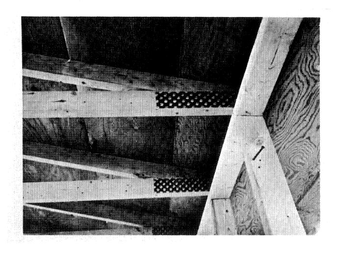
Figure 4-18. This photograph shows the truss connectors used on the Mark IV house in 1964.
