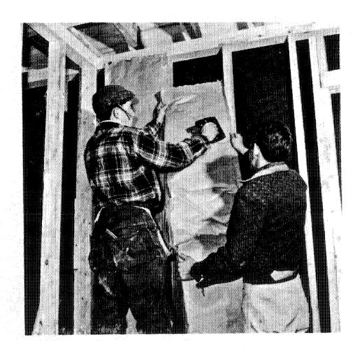
Figure 5-8. By the late 1950s, glass fibre batts stapled between the stude had become a standard type of insulation. Photograph dated 1959.
