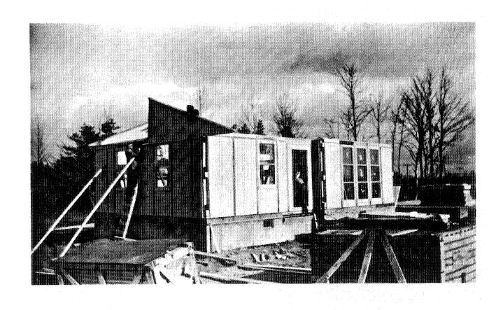
Figure 4-8. The Riley Newsum house, a prefabricated house manufactured by a British firm, was tested by CMHC at Ajax Ontario, in 1952.
