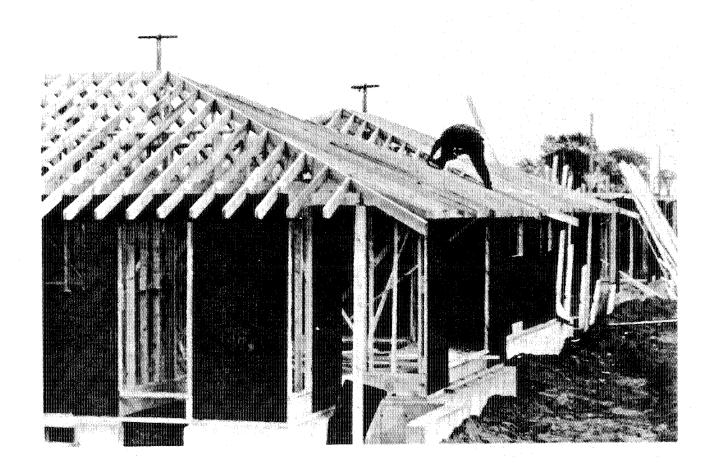
Figure 4-4. Traditionally constructed rafters, as on this Ottawa house, were labour intensive to build. Photograph not dated, probably late 1950s.
