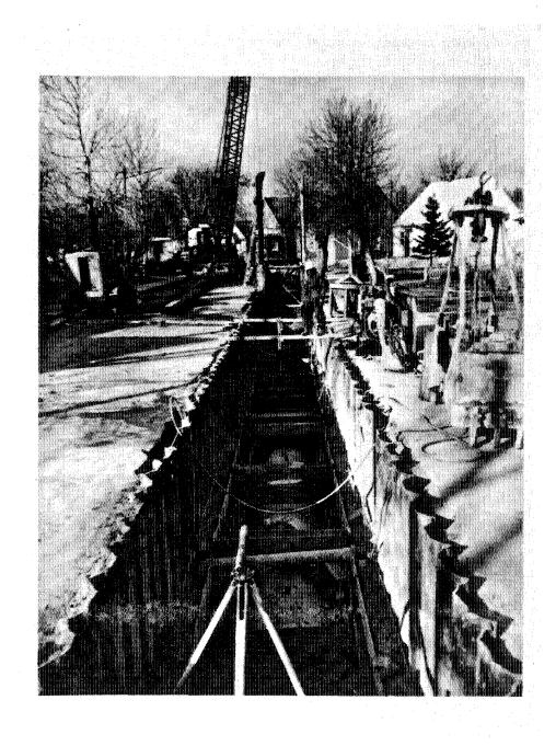
Figure 6-1. Modern urban sewage and water systems were complex and expensive. This photograph shows installation of storm sewers in Thunder Bay, Ontario. Not dated.
