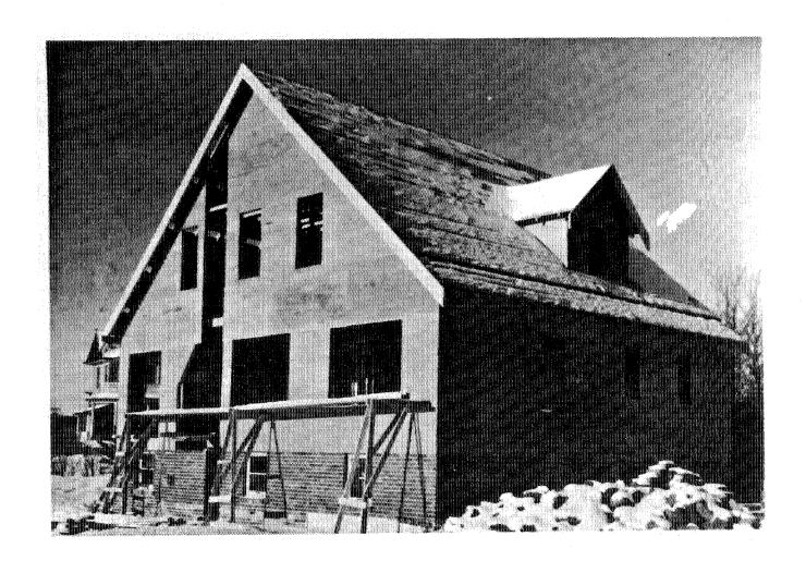
Figure 4-16. This photograph of the Muttart's house in Edmonton in 1938 shows an early use of plywood for sheathing. Following World War II, such use of plywood came into wide use.
