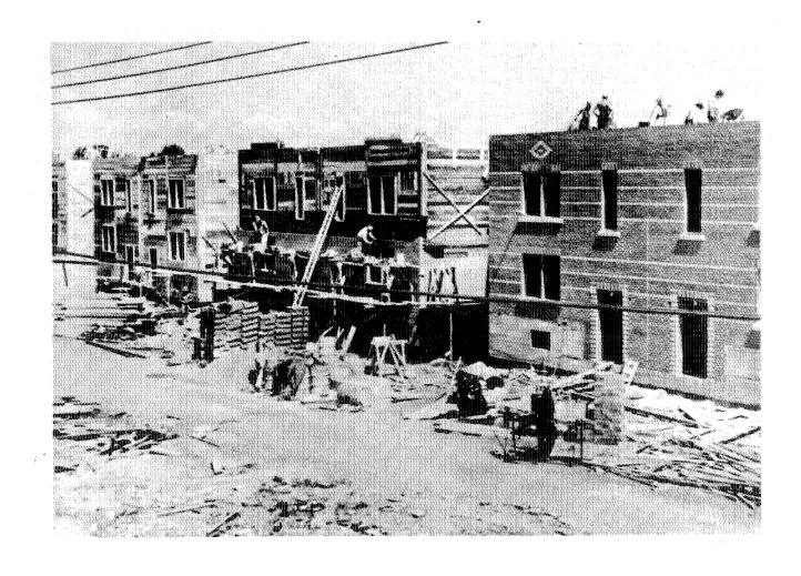
Figure 4-1. These Montreal apartments utilized Madrier construction covered with brick veneer. Not dated.
