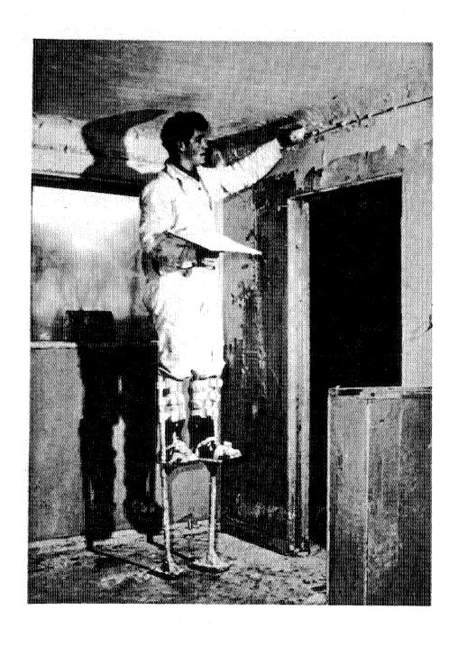
Figure 4-21. Plastering was highly skilled and labour intensive work. Photograph not dated, but probably mid 1950s.
