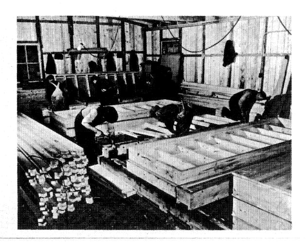
Figure 1-4. During World War II, prefabrication was used to reduce construction time. This photograph shows construction of house component parts in Halifax in 1941 for the DHAA.
