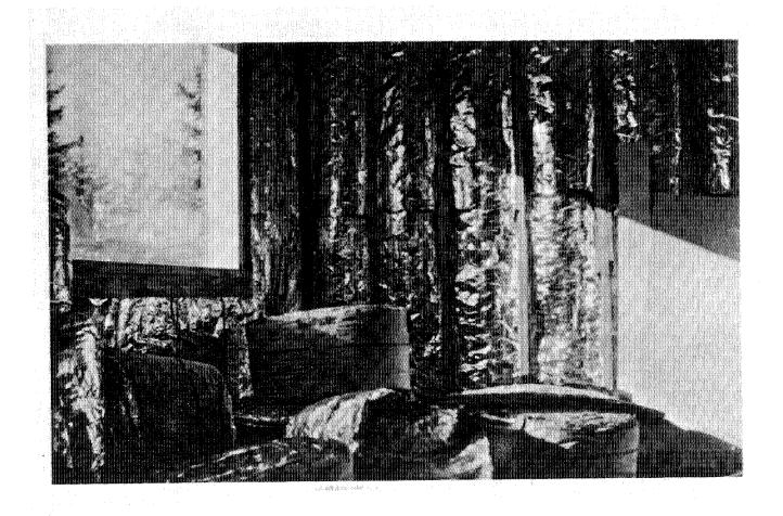
Figure 5-7. Such reflective types of insulation proved to be unsuitable in some parts of Canada. Photograph not dated.
