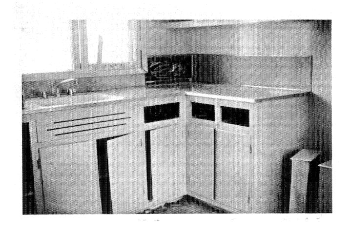
Figure 4-13. Traditionally, kitchen cabinets were built on site by carpenters, such as these ones in Capetown, New Brunswick in 1959.
