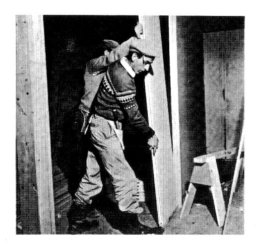
Figure 4-25. This photograph shows workers fitting together the interior partitions in the Mark III house.
