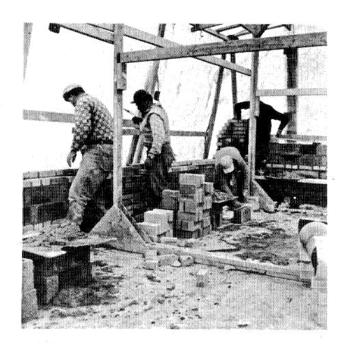
Figure 5-1. Enclosing work sites with polyethylene helped shelter workers from the cold and permitted construction throughout the year. Photograph not dated.
