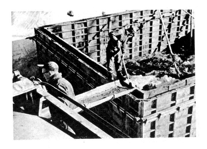
Figure 5-5. Reusable plywood forms offered one method of increasing efficiency when constructing concrete basements.
