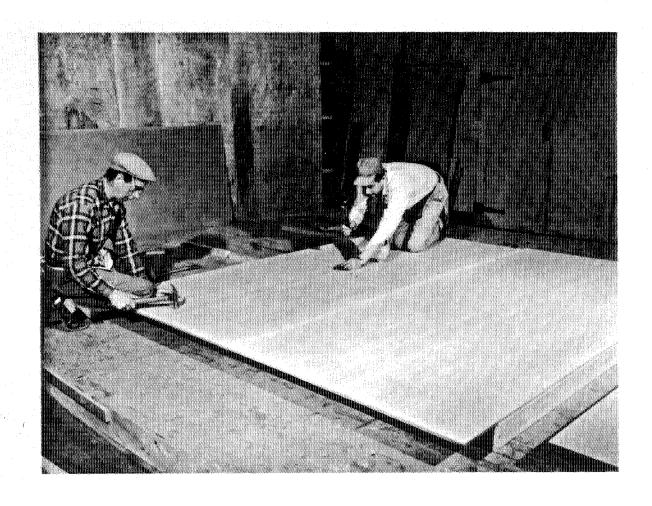
Figure 4-20. The floor of the Mark III house used stressed skin panels.
