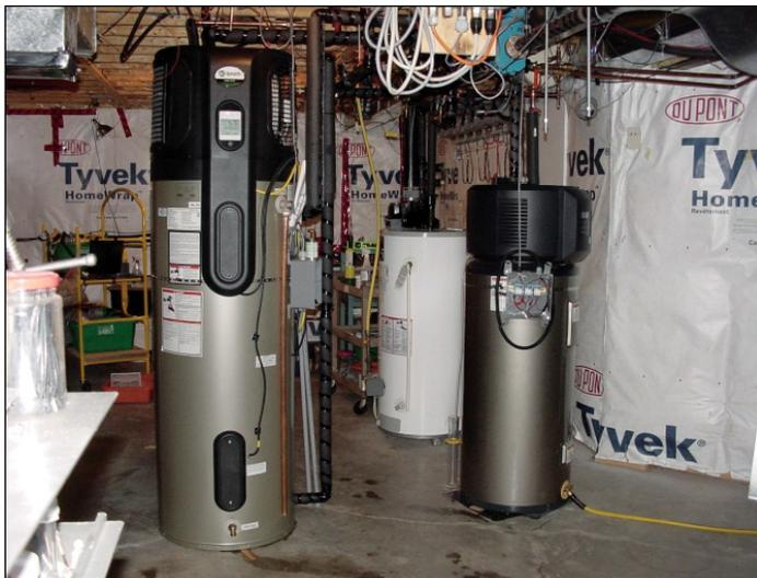
**Figure 1** Heat pump water heaters installed in the basement of the CCHT experimental house. (Left: heat pump water heater A – 80 U.S. gal./303 L, Right: Heat pump water heater B – 50 U.S. gal./189 L)
