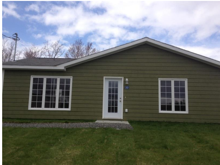
Photo: CMHC provides support for new affordable housing units on reserve (Membertou First Nation, Nova Scotia).
