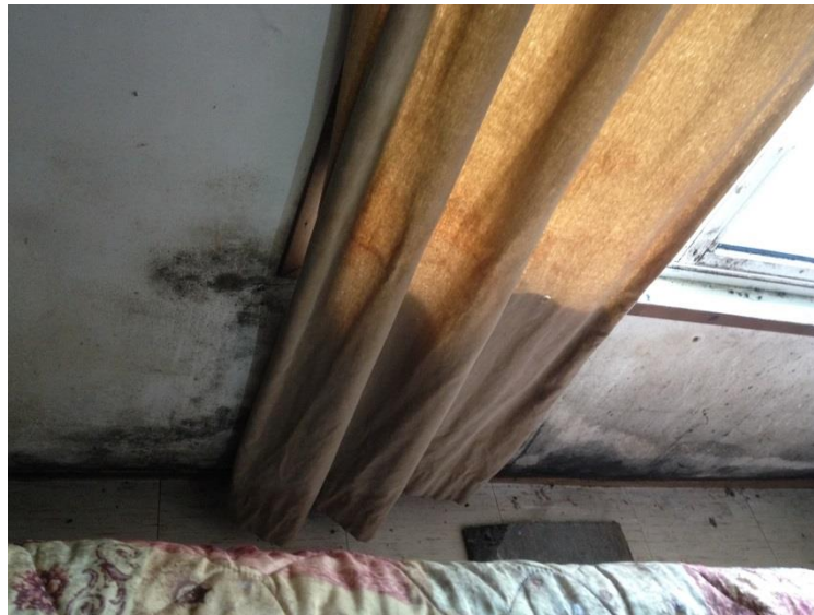
Photo: Mould in a bedroom shared by several children. (Sandy Lake First Nation, Ontario)
