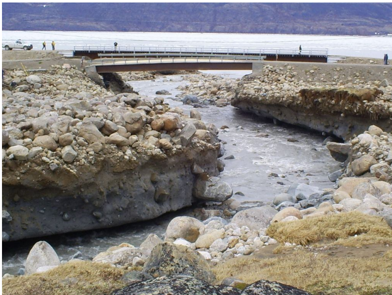
Figure 19. Photo of the impact of thermal erosion on permafrost terrain in Nunavut. This hazard was partly responsible for the destruction of the bridge in Pangnirtung. Photo credit: Hamlet of Pangnirtung.
