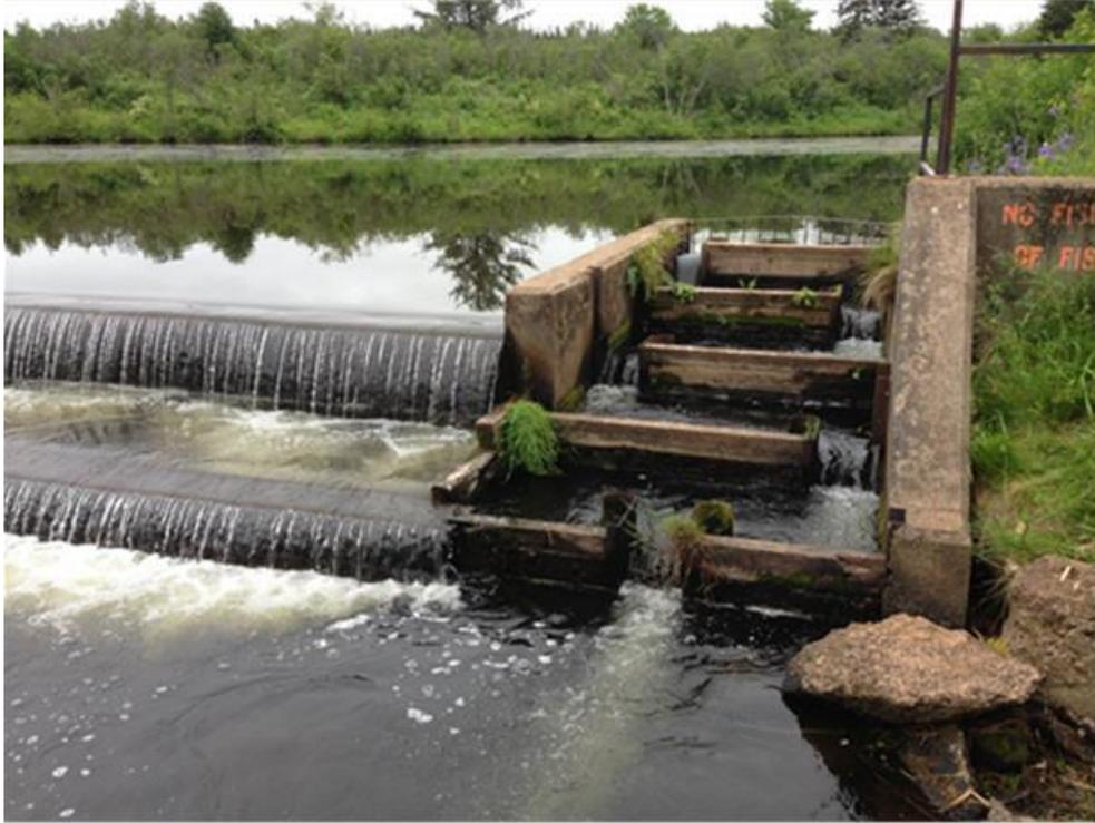
*Figure 4. View looking upstream at a small 4-cell pool-and-weir fishway with a slope of 13.1% and weir drop heights ranging from 0.08-0.21 m located on the Hillsborough River, Cherry Hill, Prince Edward Island. Photo by Sean Landsman.*
