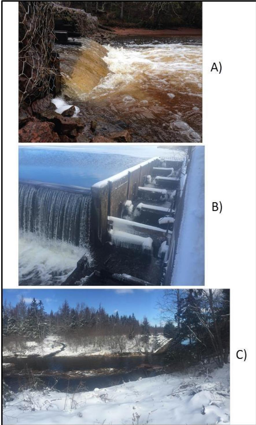
Figure 2. Side profile (A) of the outlet of a box culvert (24.2 m long, 1.4% slope) at the head-of-tide on the Glenfinnan River, Prince Edward Island Canada. The photo was taken on a low tide and shows a drop of 0.3-0.5 m to the holding pool below the culvert. Also shown are the pool-and-weir (B) and nature-like bypass channel (C; far shoreline) fishways. Photos by Sean Landsman.
