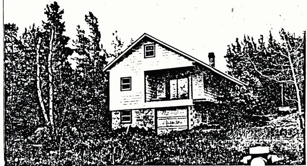
Above-left: Major repairs required, and overcrowded conditions.
