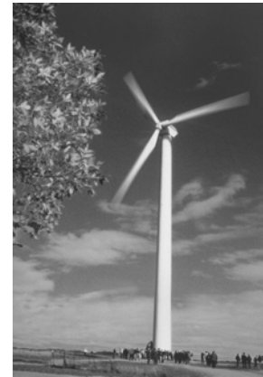
Wind turbine at Kincardine, Ontario (photo courtesy of Paul Gipe)
