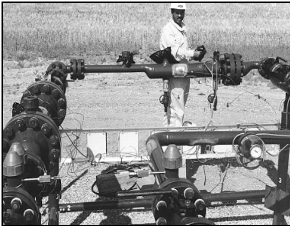
Corrosion measurement in the field
