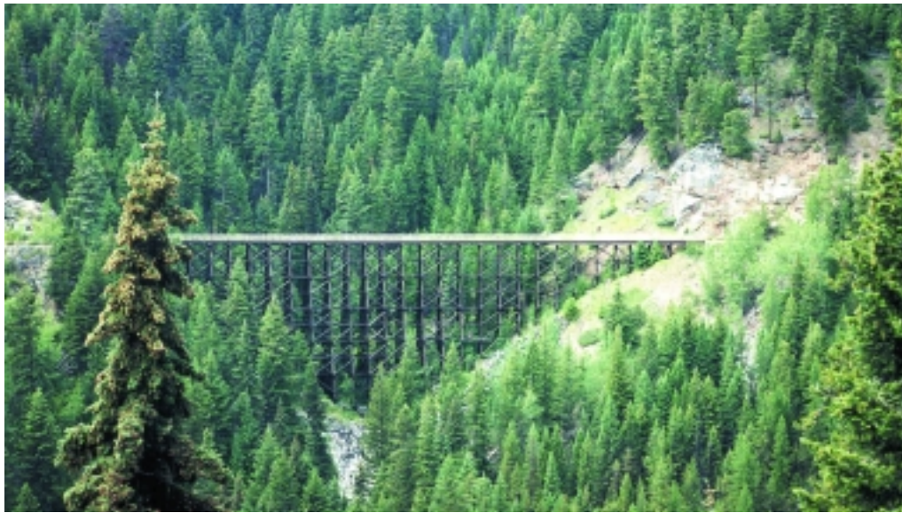
The Chrysler Trestle, Kettle Valley Trail.
