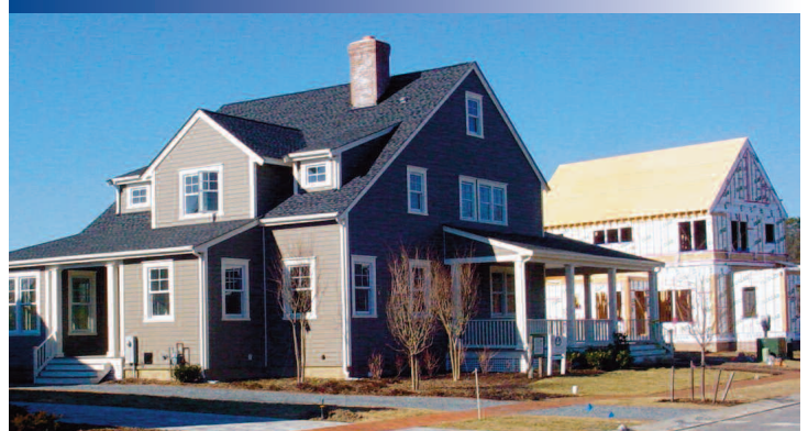
A DAC International home in Easton, Maryland.
