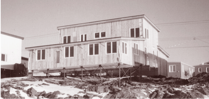
Steenberg Construction's bed and breakfast in Iqaluit, Nunavut—a commercial application of "Health House" techniques in northern Canada.
