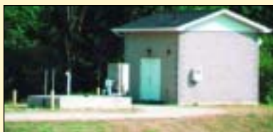
Sewage Pumping Station
