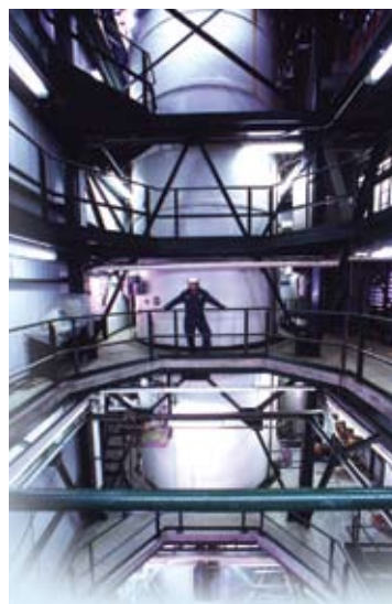
logen Corporation's cellulose ethanol demonstration facility, Ottawa.
