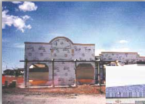
Moccasin Flats Plaza during construction
