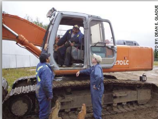
Construction crews working in the Wabasca area.
