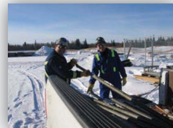
Seven Lakes employees unloading pipe
