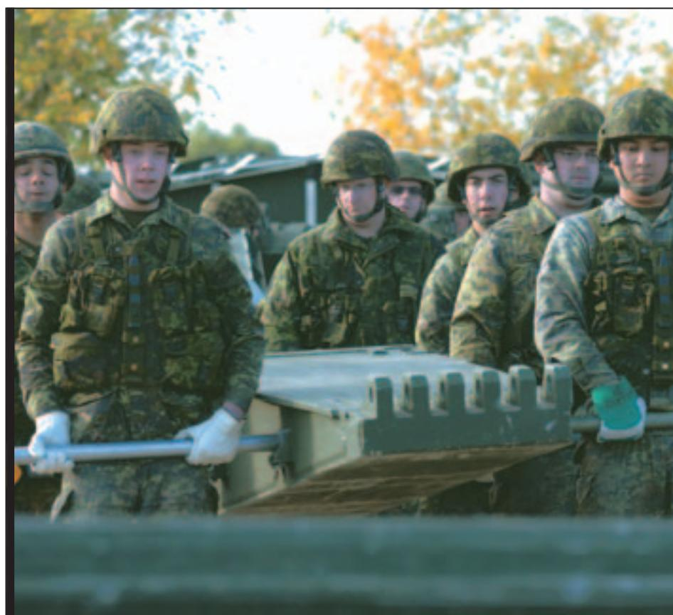
Muscling around the bulky components of the medium girder bridge, members of 31, 32 and 33 Combat Engineer Regiments assemble a medium girder bridge as part of a training exercise.
