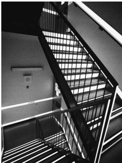
PLM lights the way in this high-rise stairwell.
