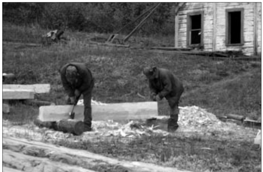
Hewing logs for the Cadzow House
