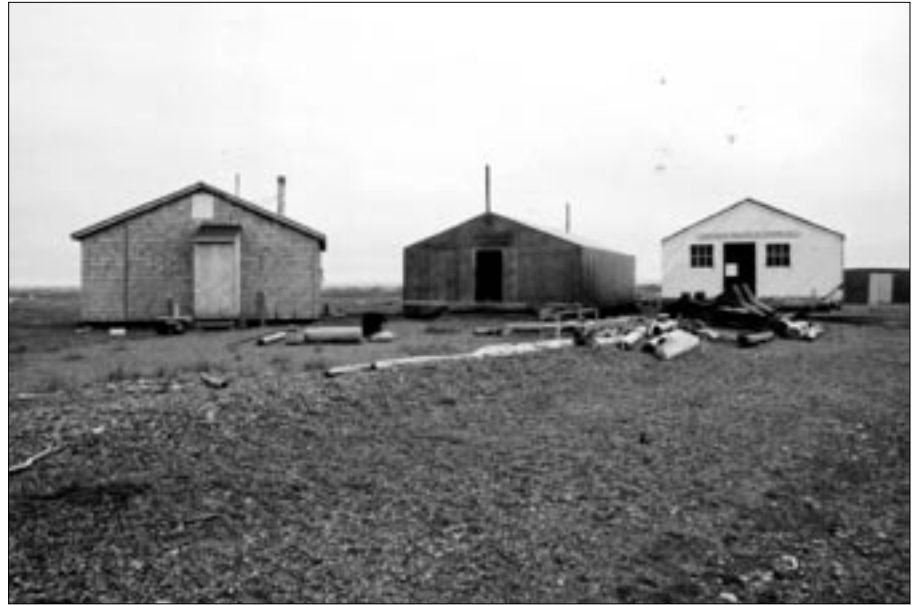
Relocated Herschel Island buildings (left to right – hunters and travellers cabin; Canada Customs Warehouse; Northern Whaling and Trading Co. Store)
