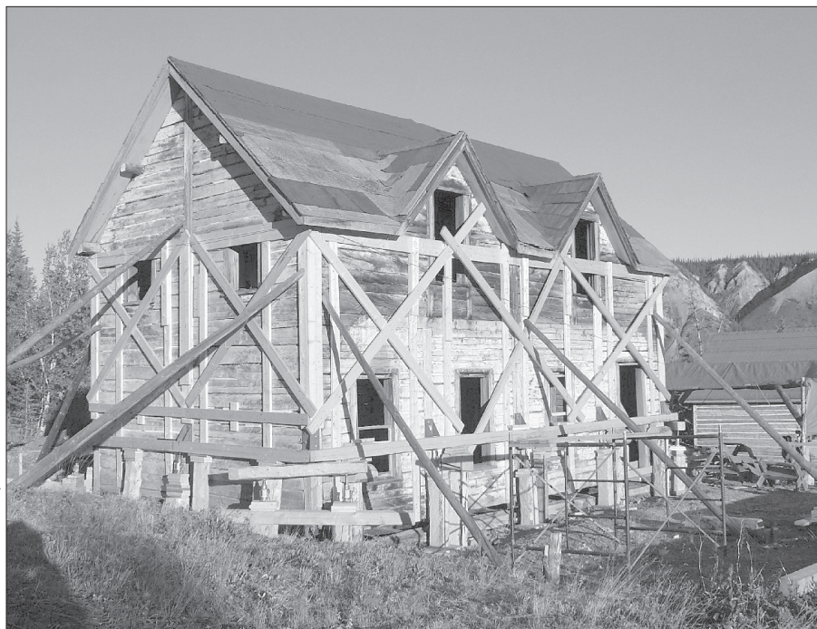
Cadzow House braced for lifting.
