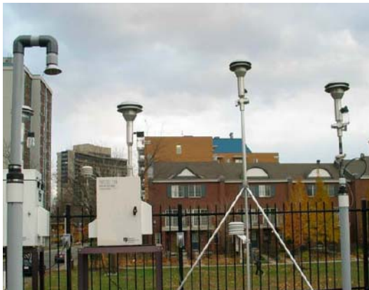
Figure 3 An air quality monitoring station
